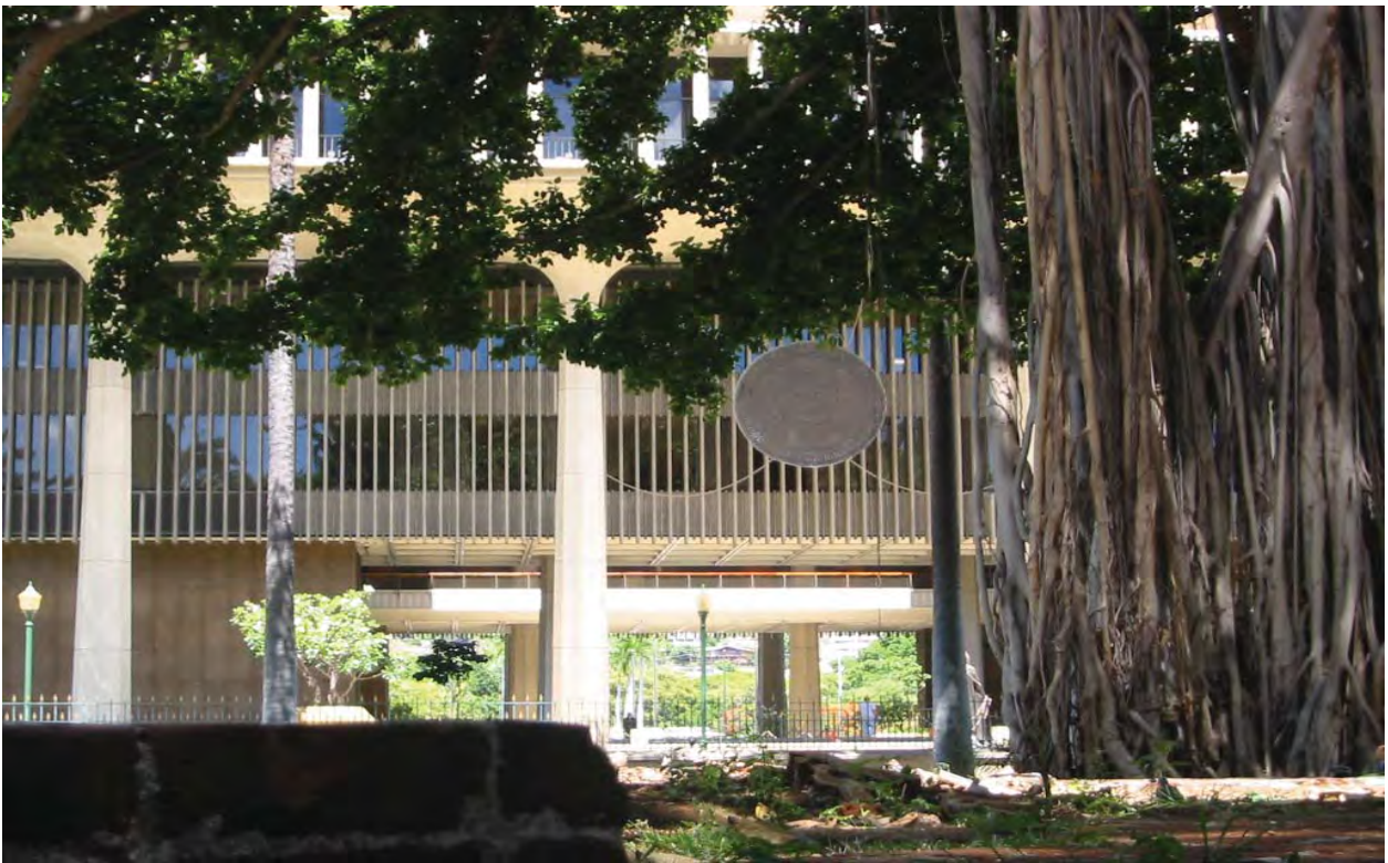
Figure 1 —An enormous fig tree graces the grounds of Hawai'i's state capitol in Honolulu. Public trees in Honolulu provide great benefits, improving air quality, sequestering carbon dioxide, reducing stormwater runoff and beautifying the city. The trees of Honolulu return $2.98 in benefits for every $1 spent on tree care.
